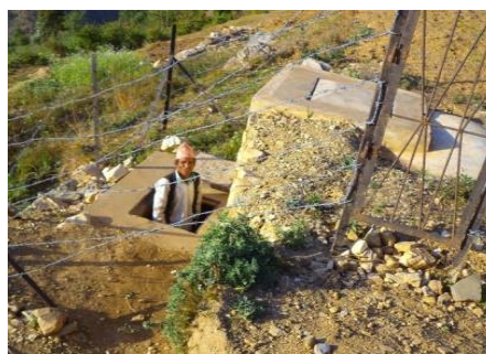
Photo 12 : GFS maintenance Jajarkot
